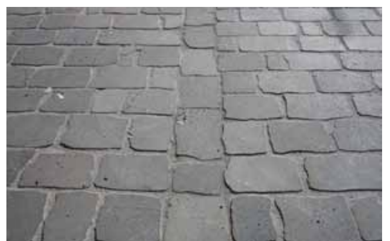
Sawn bluestone paving to property frontages
